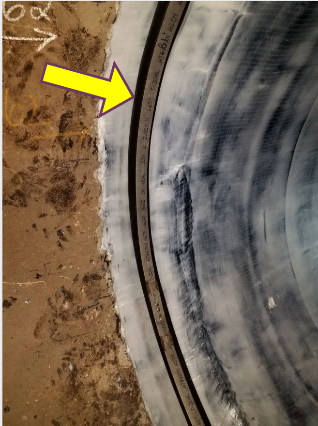
Termination ring at joint of repaired pipe
