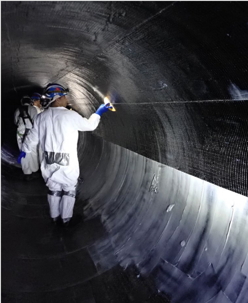
Installation of Carbon Fiber and Thickened Epoxy
