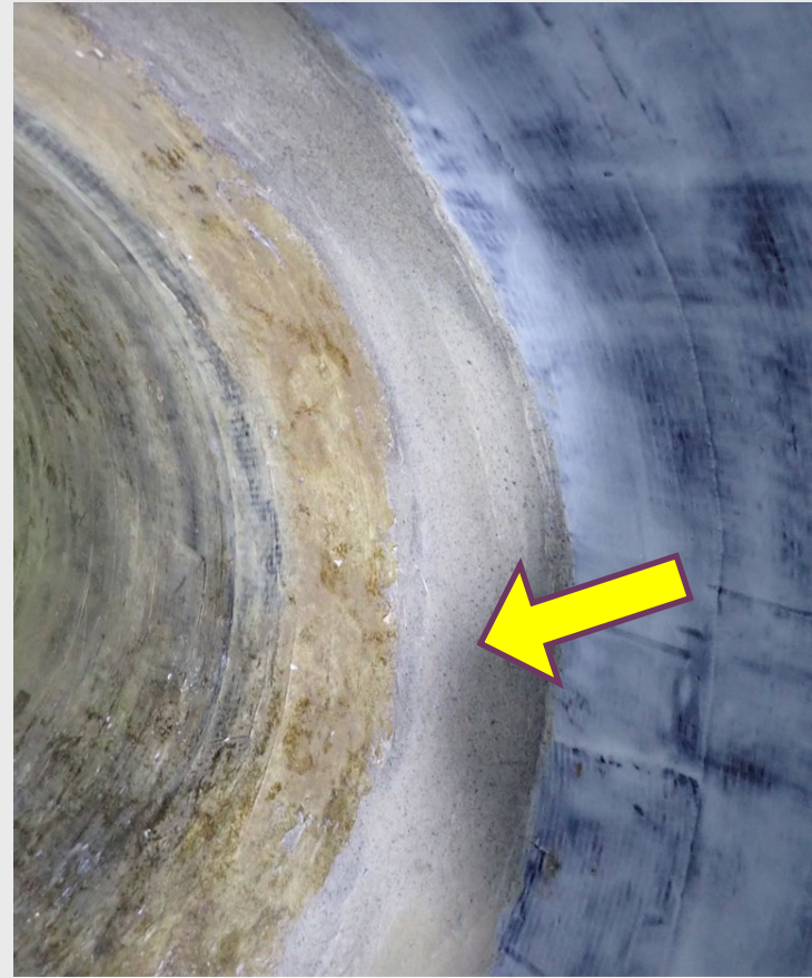
Epoxy cement mortar covering termination ring
