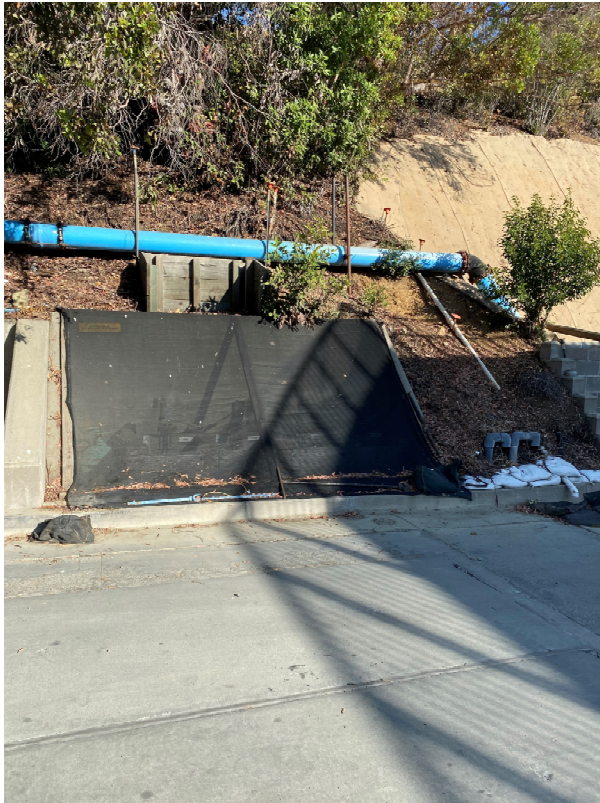
Concrete Pipe Support Work – Before and After
