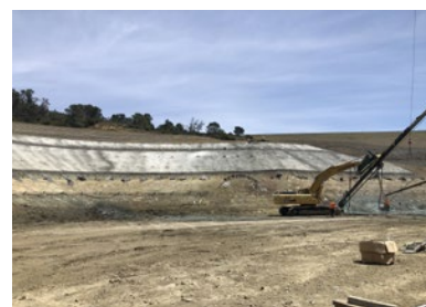
Crew installing soil nails to reinforce the hillside surrounding the Diversion Portal area.
