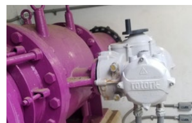
Plunger Valve at Main Avenue Ponds Vault.
