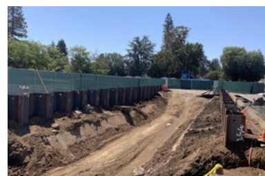
Installed sheet piles at Hale Creek
