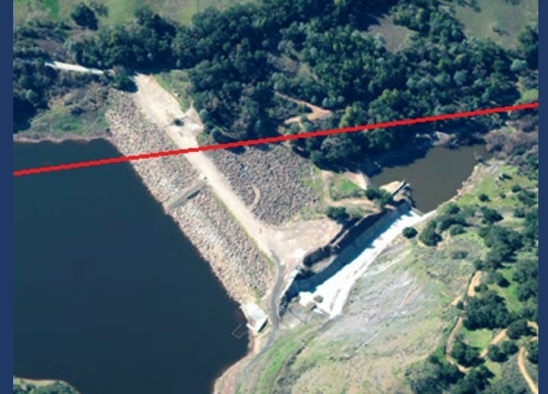
Calaveras Fault crossing embankment
