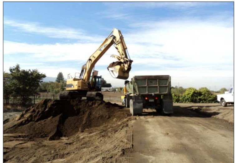
Sludge pond sediment removal at Santa Teresa Water Treatment Plant
