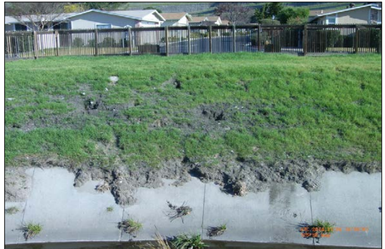
View of damage caused by burrowing animals along Canoas Creek in the Guadalupe Watershed
