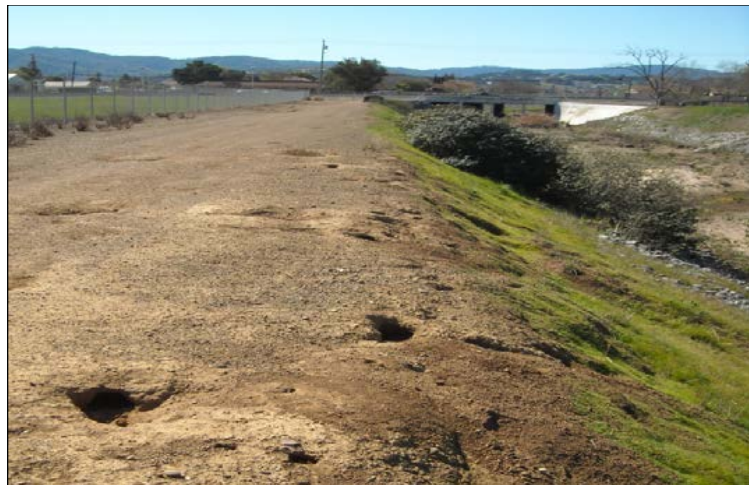
View of damage caused by burrowing animals along West Branch of Llagas Creek in the Uvas/Llagas Watershed
