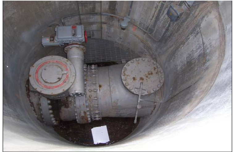
A typical line valve assembly to be rehabilitated
