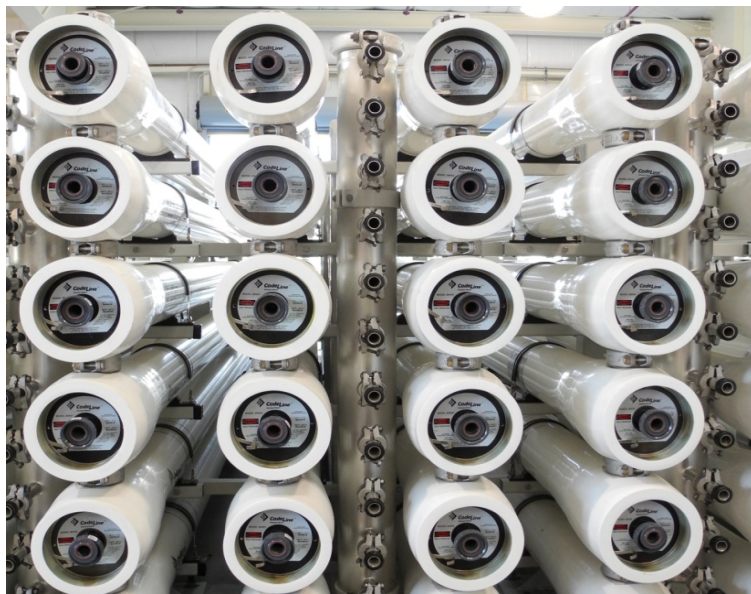
Reverse osmosis membranes used for water purification
