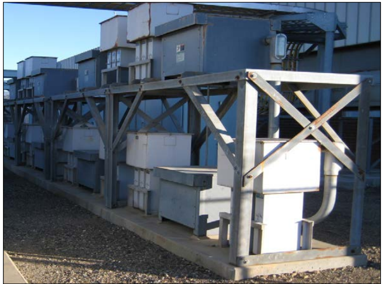
ASD Motors at the Coyote Pumping Plant
