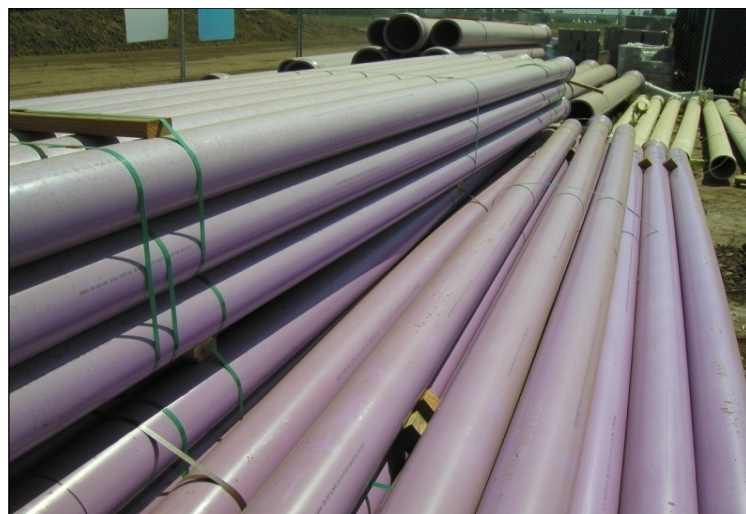
Recycled water purple pipeline waiting to be laid during construction of Immediate Term project
