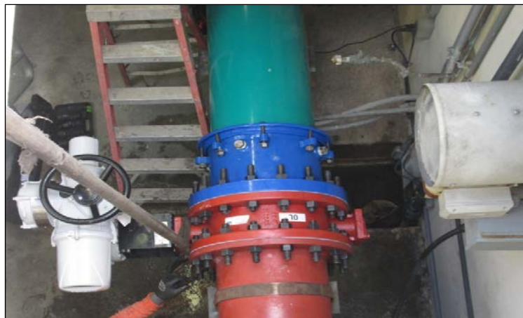
A typical rehabilitated line valve assembly
