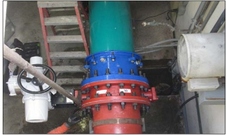
A typical rehabilitated line valve assembly
