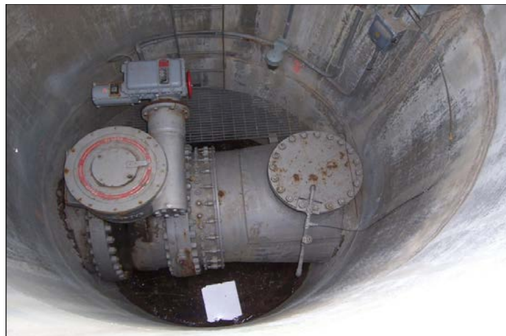
A typical line valve assembly to be rehabilitated
