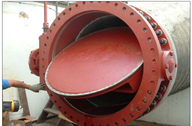
Small Capital projects at treated water transmission facilities, similar to this new valve installation in the Piedmont Line Valve Vault, will be done, per the asset management plan.
