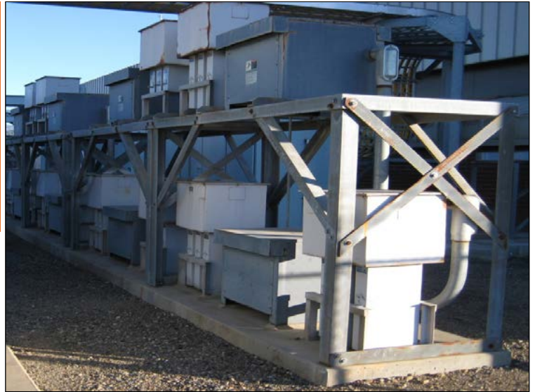
ASD Motors at the Coyote Pumping Plant
