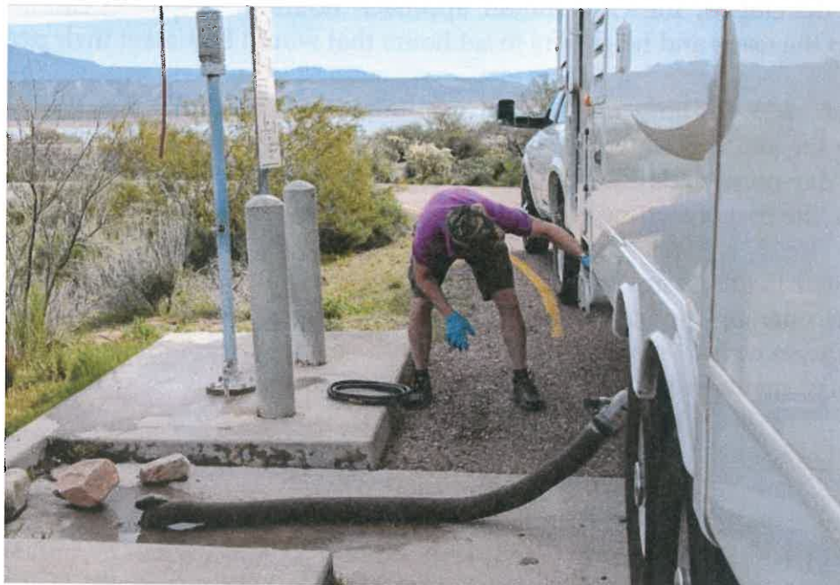
Figure 2 – Dump Station with At-Grade Sewer Connection
