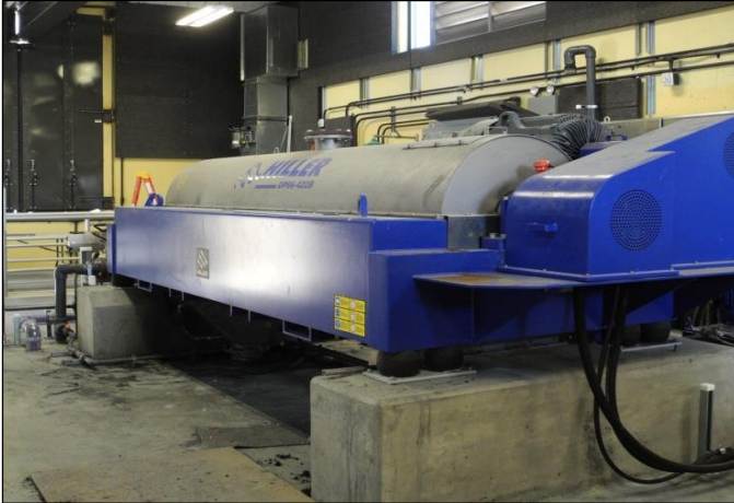
Centrifuge for mechanical dewatering of sludge
