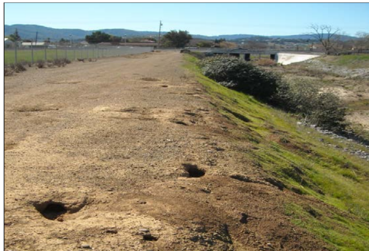
View of damage caused by burrowing animals along West Branch of Llagas Creek in the Uvas/Llagas Watershed
