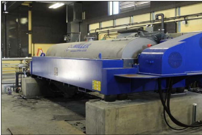
Centrifuge for mechanical dewatering of sludge
