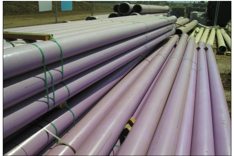
Recycled water purple pipeline waiting to be laid during construction of Immediate Term project
