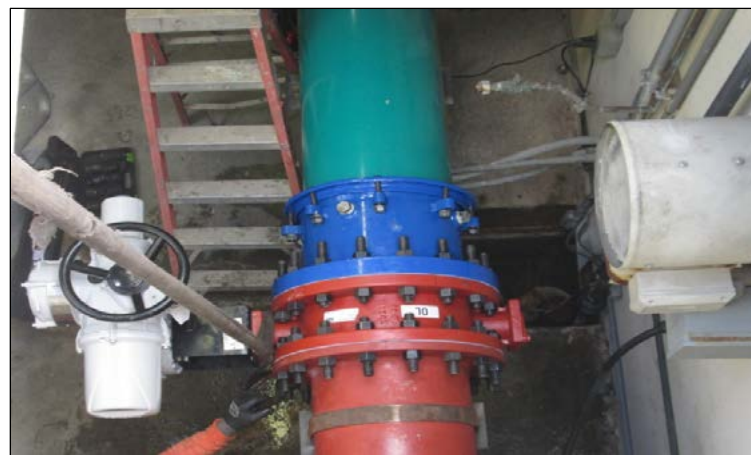
A typical rehabilitated line valve assembly
