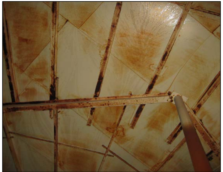
Active corrosion of the rafters and rafter support
