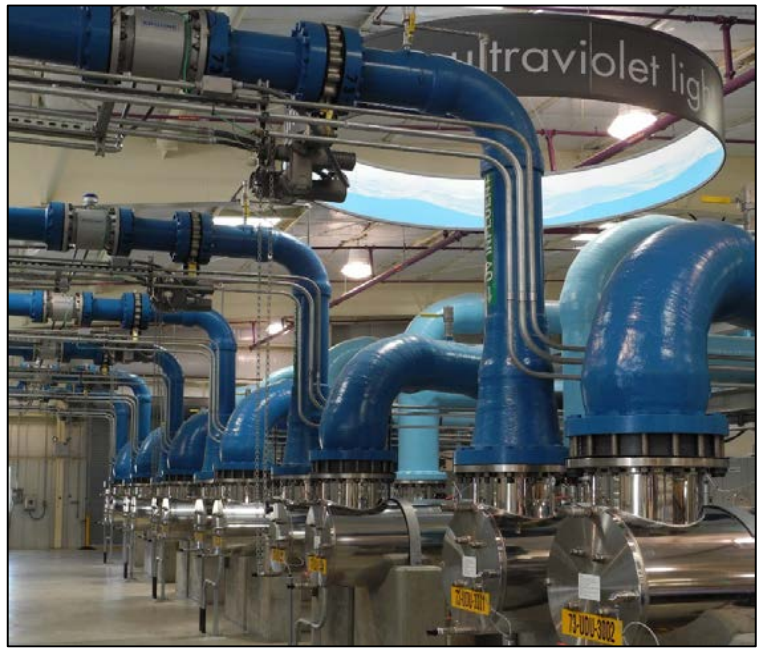
Water is exposed to ultraviolet light in purification process
