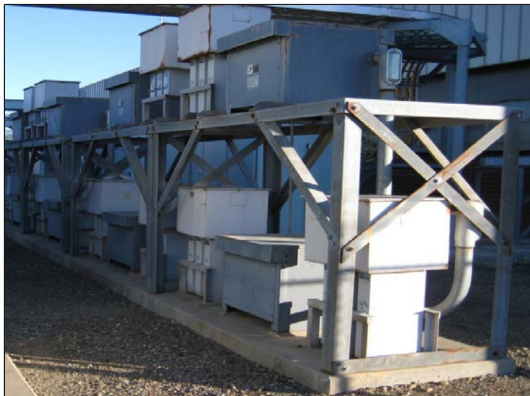
ASD Motors at the Coyote Pumping Plant
