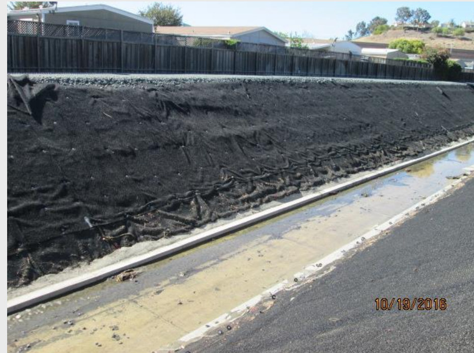
Canoas Creek – Erosion Control Fabric
