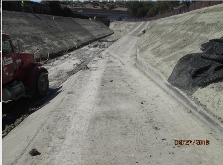
Canoas Creek – Finished Embankment Slopes
