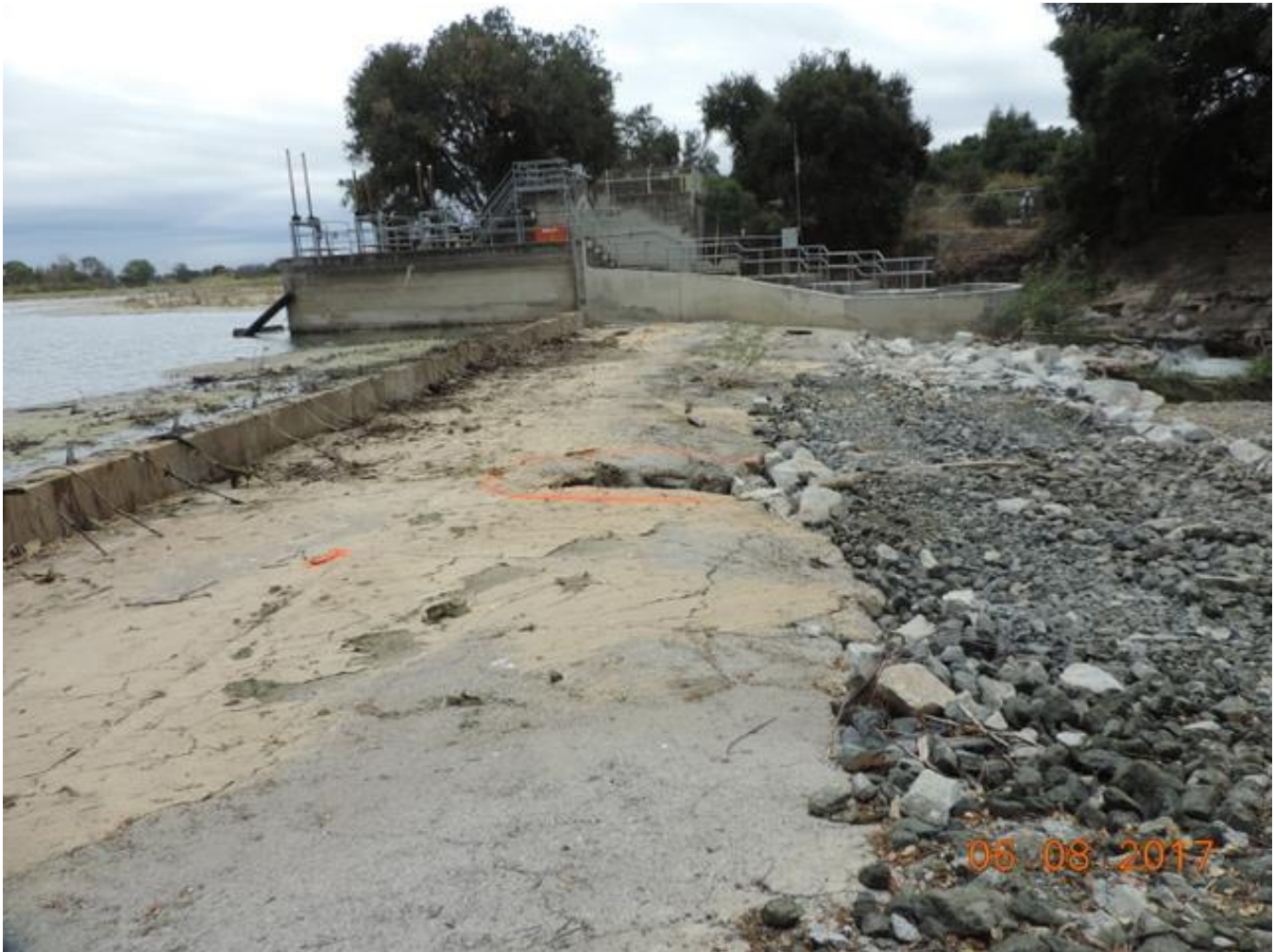
Photo 3: Dewatered site showing damaged apron and downstream buttress – June 2017
