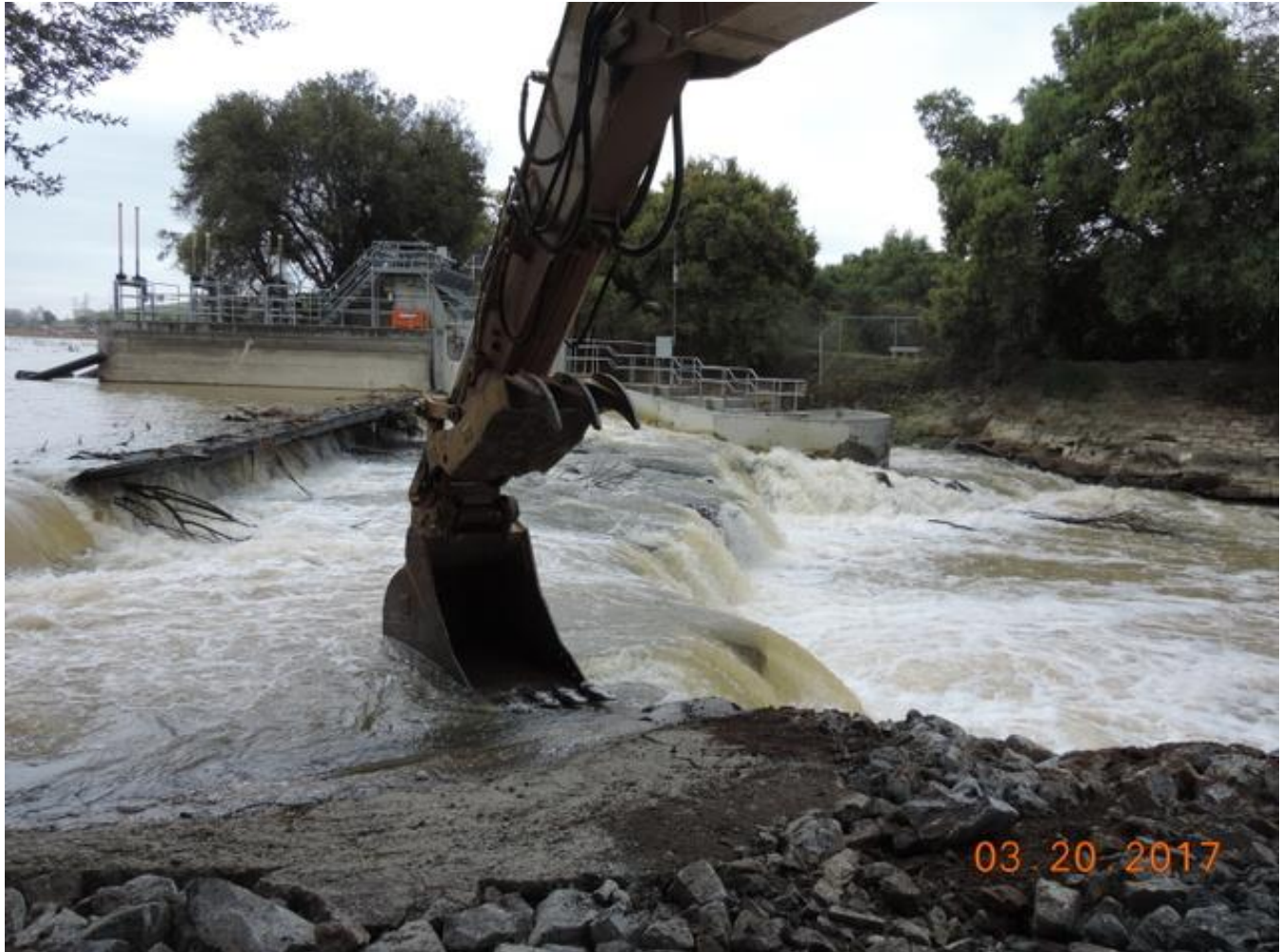
Photo 2: Emergency work to buttress downstream side of dam – March 2017
