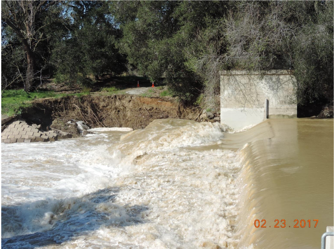
Photo 1: High flows and erosion caused by February storms – February 2017
