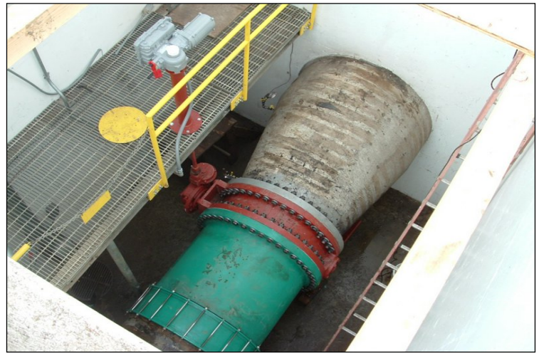
New line valves, actuators, and vaults similar to this will be installed along the East, West, and Snell pipelines
