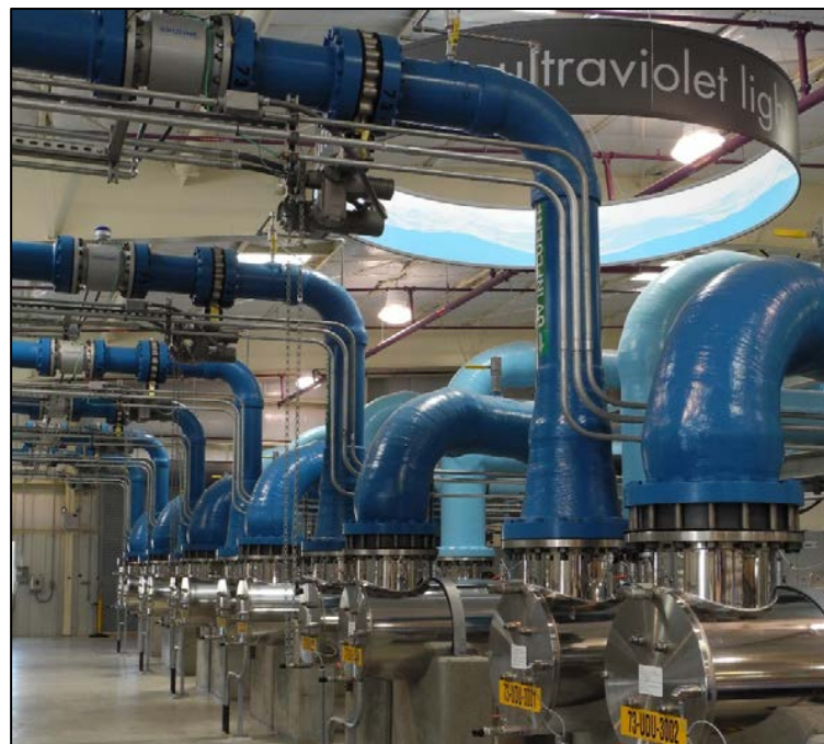
Water is exposed to ultraviolet light in purification process
