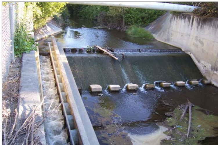
Example of a fish ladder to be modified or reconstructed for better fish passage
