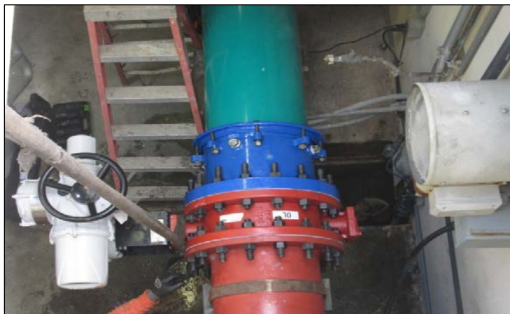
A typical rehabilitated line valve assembly
