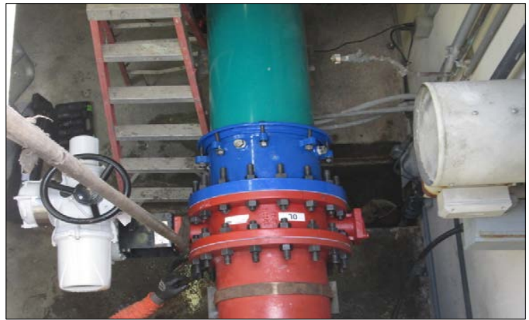
A typical rehabilitated line valve assembly
