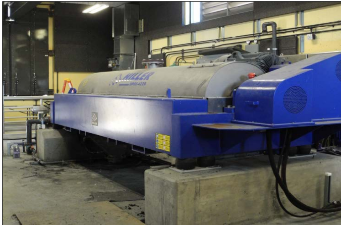
Centrifuge for mechanical dewatering of sludge
