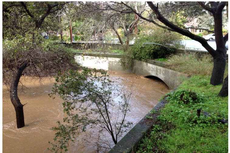
Upstream face of Pope/Chaucer Street with water surface approximately 2 feet below the soffit
