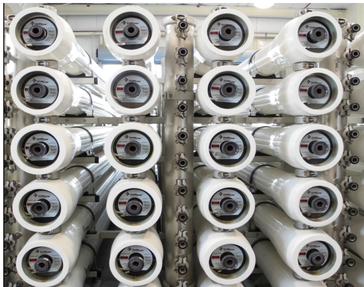
Reverse osmosis membranes used for water purification
