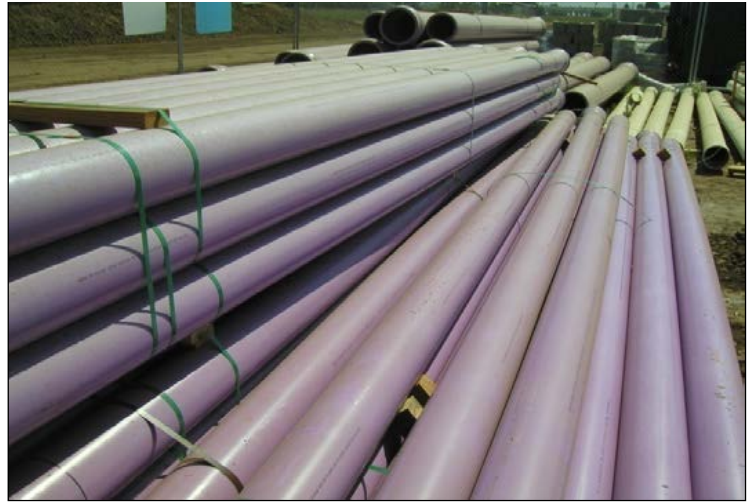
Purple recycled water pipe waiting to be laid during construction of Immediate Term project
