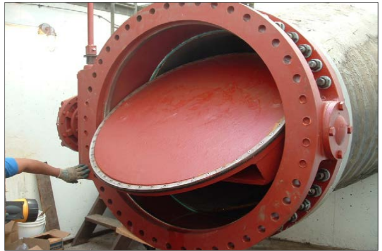
Valve installation in the Piedmont Line Valve Vault; Similar small capital projects will be carried out at treated water transmission facilities according to the asset management plan.
