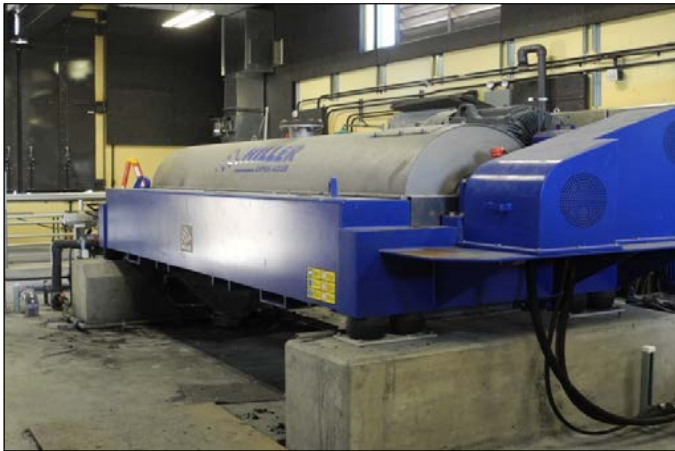
Centrifuge for mechanical dewatering of sludge
