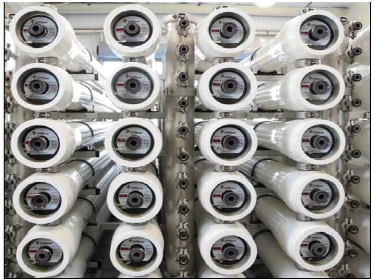
Reverse osmosis membranes used for water purification
