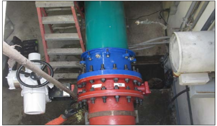
A typical rehabilitated line valve assembly
