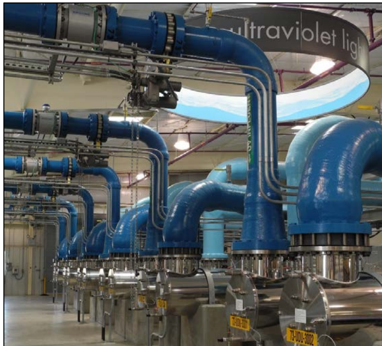
Water is exposed to ultraviolet light in the purification process
