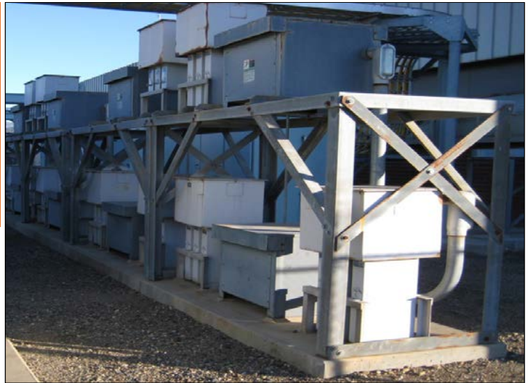
ASD motors at the Coyote Pumping Plant
