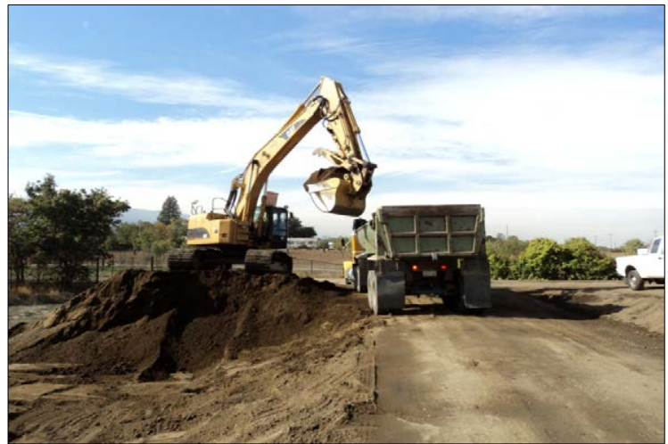
Sludge pond sediment removal at Santa Teresa Water Treatment Plant
