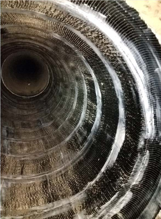
Hoop and Longitudinal Layer of Carbon Fiber
