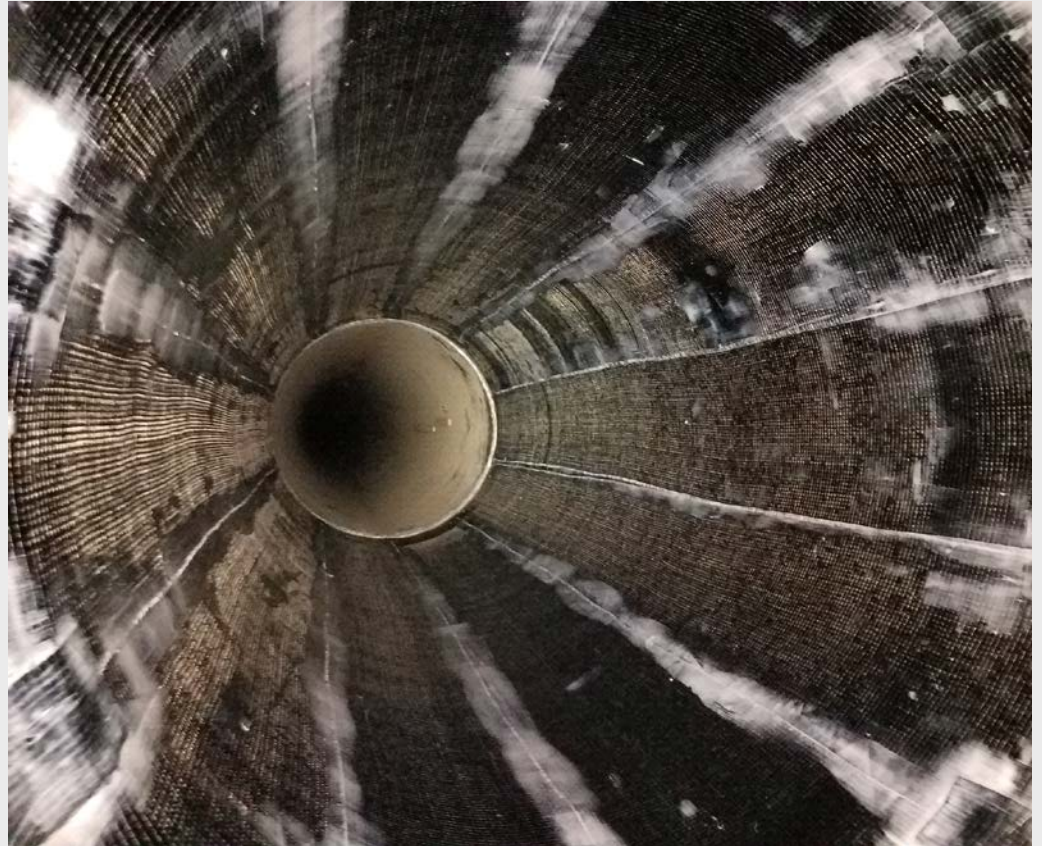
Hoop and Longitudinal Layer of Carbon Fiber
