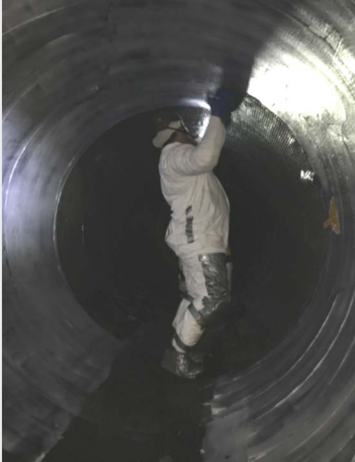
Installation of Carbon Fiber and Thickened Epoxy
