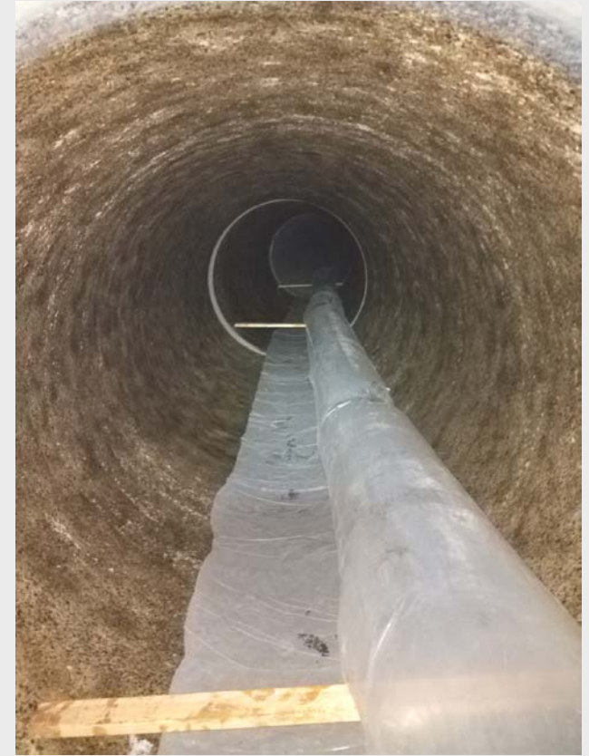
Dehumidifier and heater for installation of carbon fiber.
