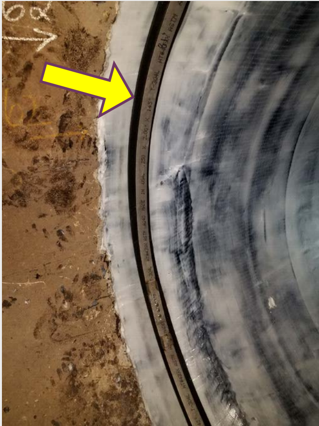
Termination ring at joint of repaired pipe
