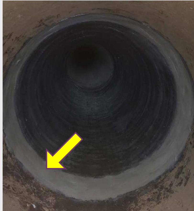
Epoxy mortar covering termination ring
