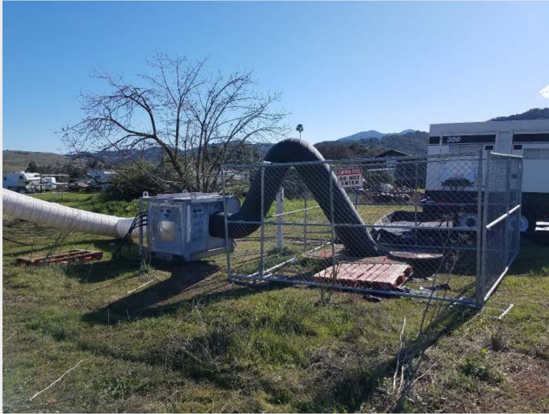
Dehumidifier and heater for installation of carbon fiber.
