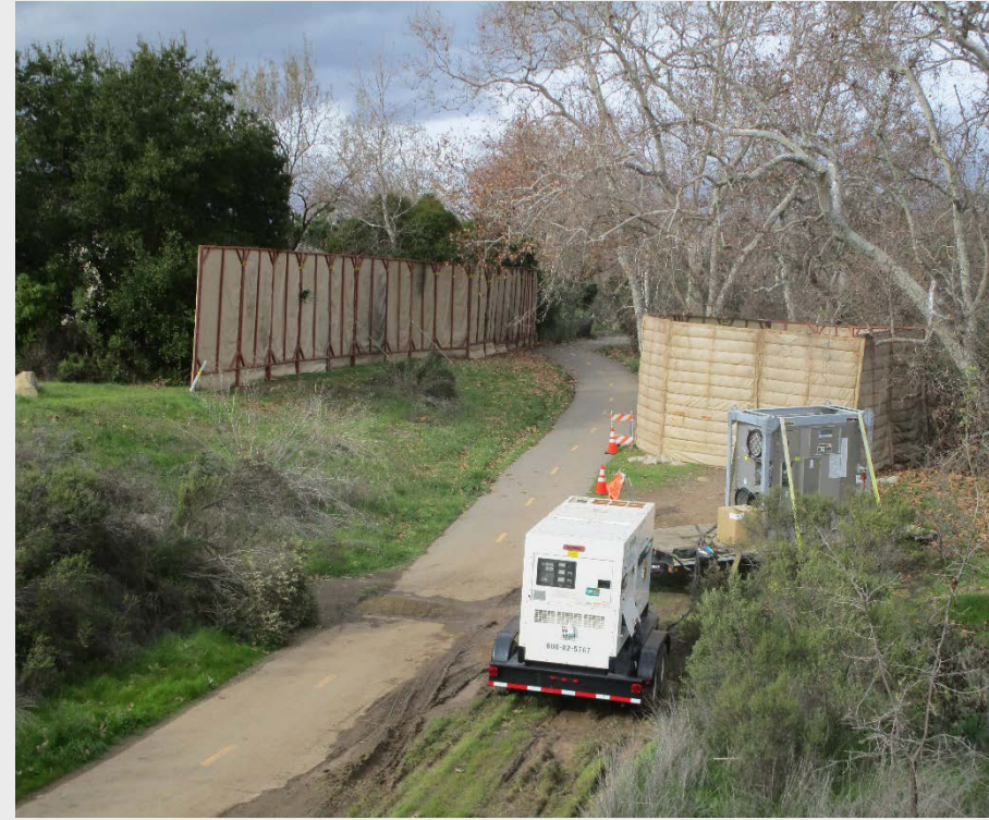
Installation of sound panels and temporary power.
