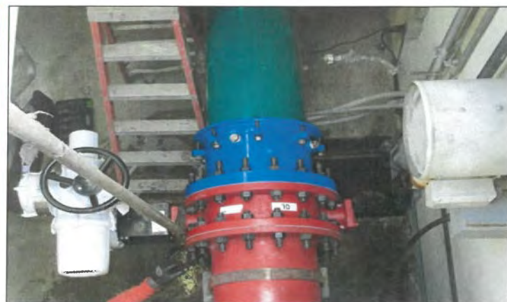
A typical rehabilitated line valve assembly
