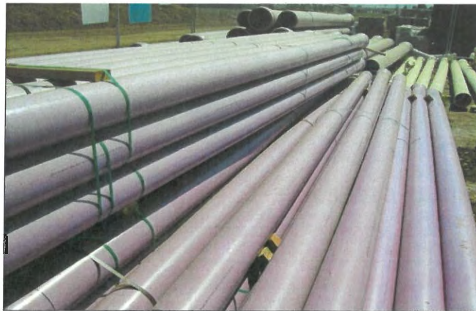
Purple recycled water pipe waiting to be laid during construction of Immediate Term project
