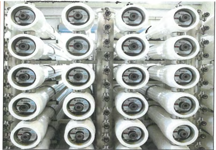
Reverse osmosis membranes used for water purification
