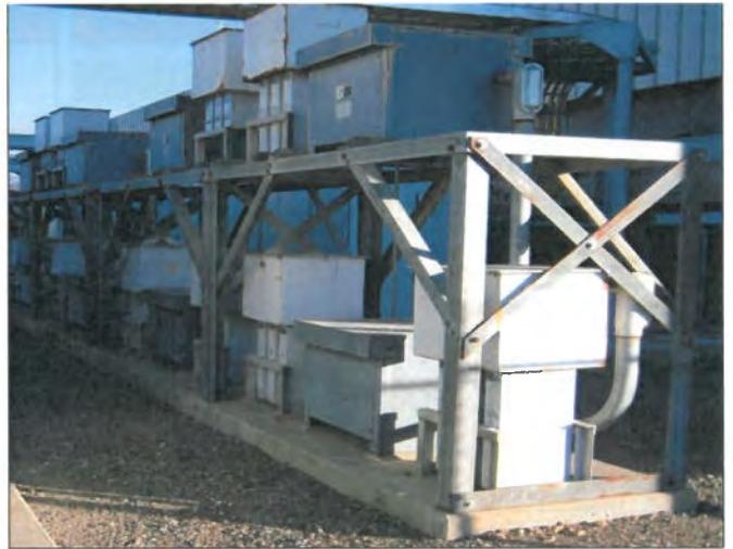
ASD motors at the Coyote Pumping Plant
