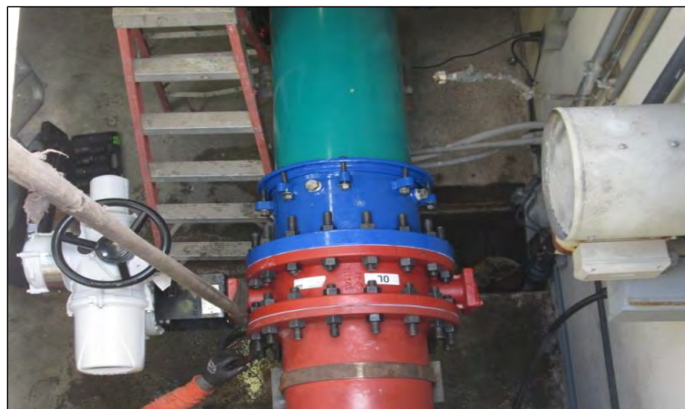
A typical rehabilitated line valve assembly
