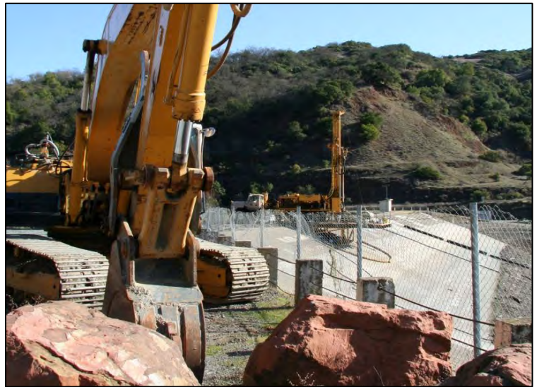
Field exploration for seismic stability evaluations
