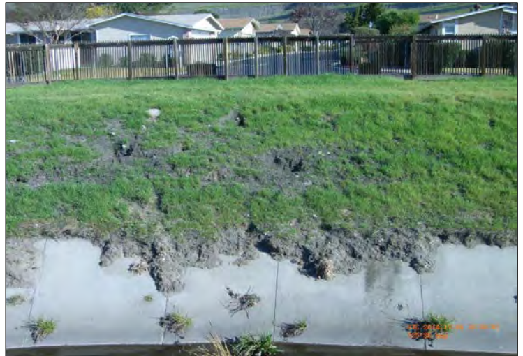
View of damage caused by burrowing animals along Canoas Creek in the Guadalupe Watershed
