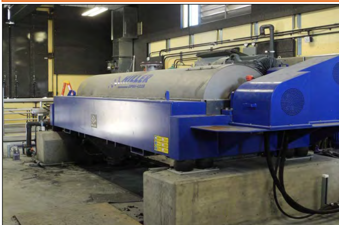
Centrifuge for mechanical dewatering of sludge
