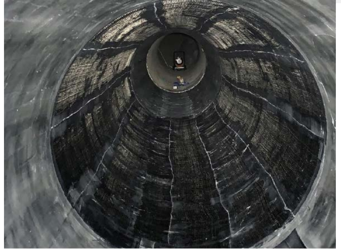
Hoop and Longitudinal Layer of Carbon Fiber
