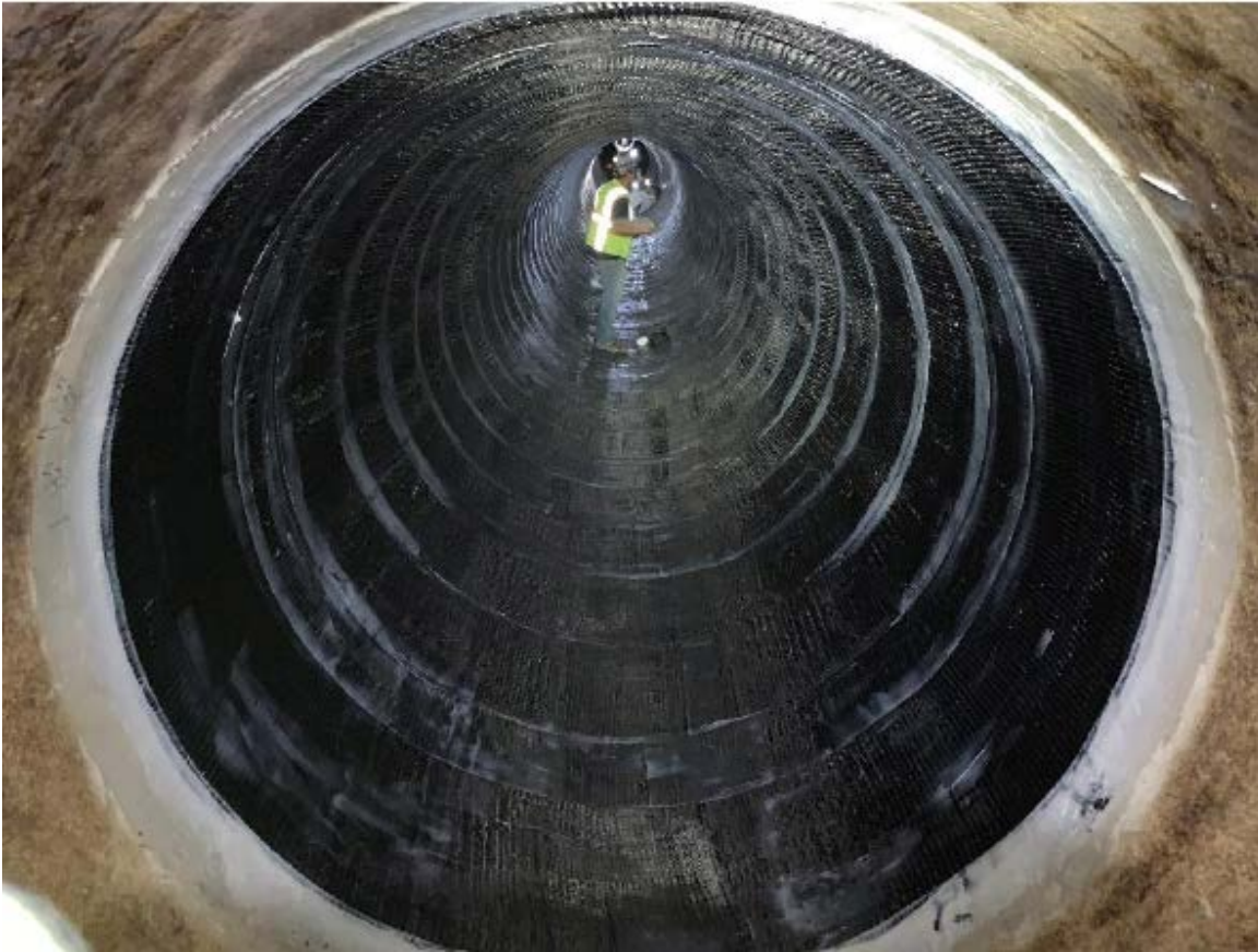
Hoop and Longitudinal Layer of Carbon Fiber
