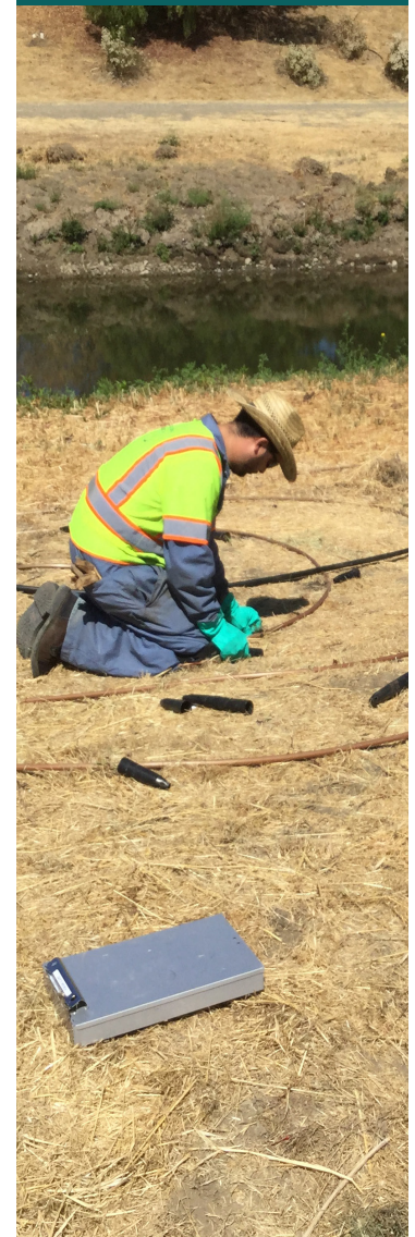
Installing irrigation in Guadalupe River
