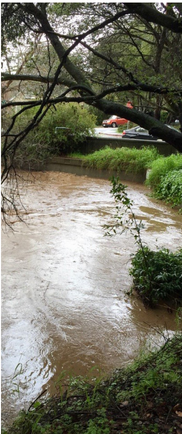
High flows under the Pope/Chaucer Street Bridge
