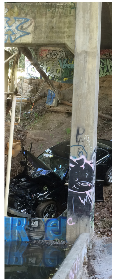
Vehicle accident at Valley Water facility.
