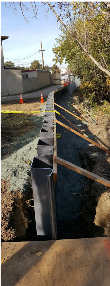
Interim floodwall and embankment along Coyote Creek in the Rock Springs community
