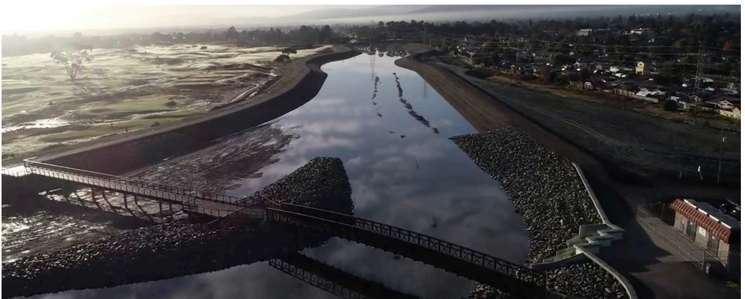
2012 Safe, Clean Water Program: Looking upstream from the Friendship Bridge at the completed portion of the San Francisquito Creek Flood Protection Project from S.F. Bay to Highway 101
