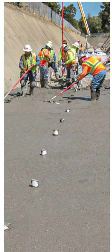
San Tomas erosion repair.
