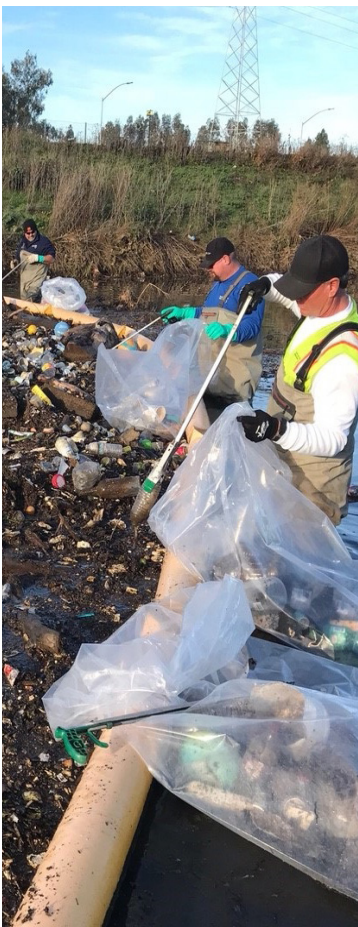
Trash boom cleaning on Lower Silver Creek.
