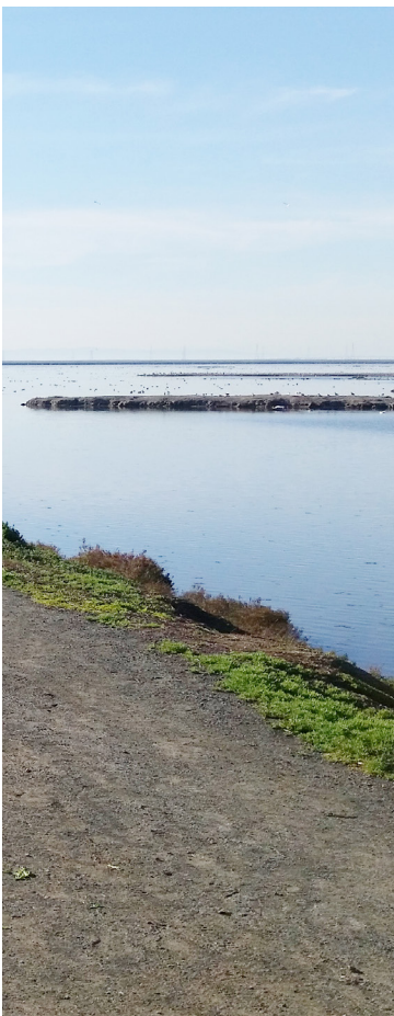
Shoreline Phase 1 levee
