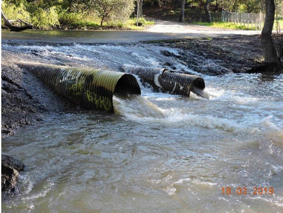
Photo 7. Singleton Road crossing at a dropping stream flow of about 140 cfs on 18 March 2019. High velocity in the culverts and the shallow flow over the apron probably prevented adult steelhead upstream passage.
