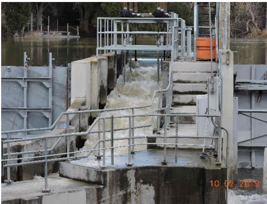
Photo 2. The fish ladder at Metcalf Dam on 10 February 2019. Despite turbulence in the ladder, it was probably passable by adult steelhead (if they successfully located the ladder in the high flows).
