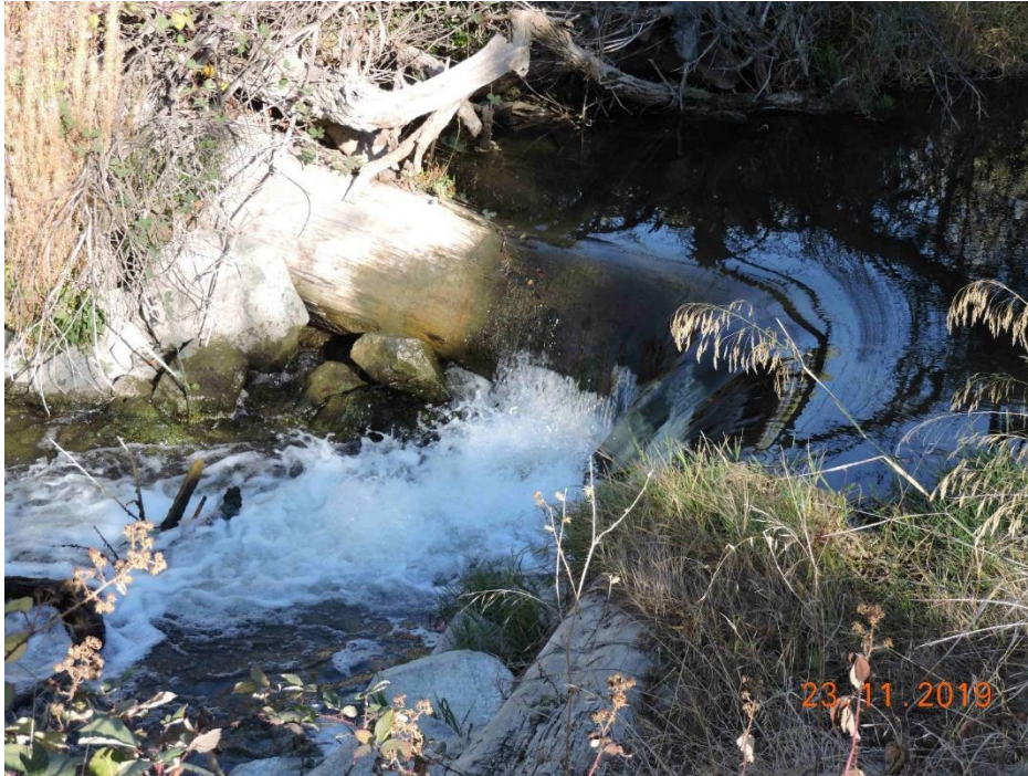
Photo 5. The stream gage weir at Coyote Ranch Road on 23 November 2019 at a flow of 13 cfs, showing the very difficult potential fish passage.
