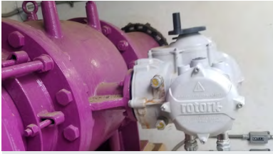
Plunger Valve at Main Avenue Ponds Vault.
