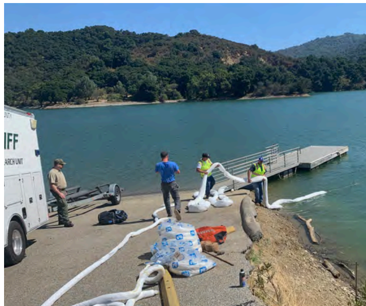
Boom deployment at Stevens Creek Reservoir.
