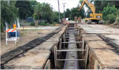
Main Ave. pipeline installation.
