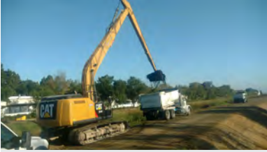
Sediment removal at Sunnyvale East Channel.
