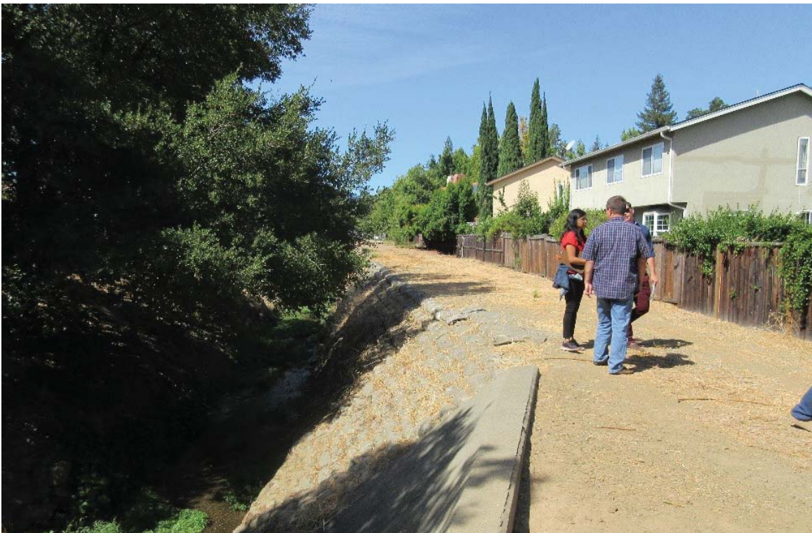
Photo 4 View of creek facing west on the north side of the creek. The trail would be placed on the existing maintenance road shown. Sacked concrete and mature oak trees can be seen within the banks of the creek.
