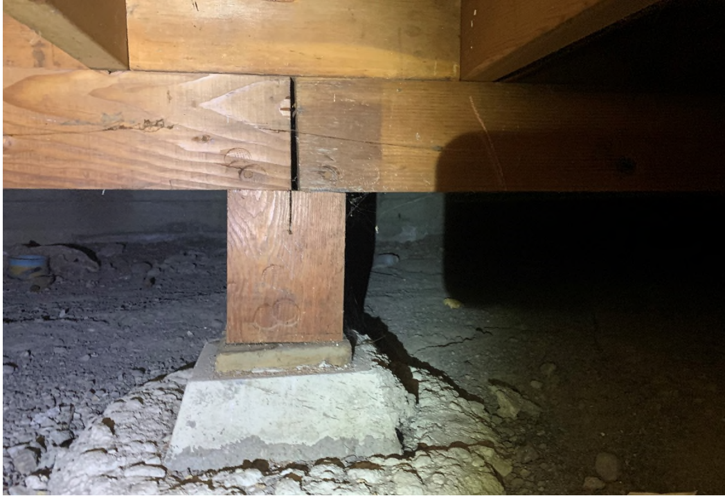
Photo No. 7: Below the home, the crawl space revealed floor framing inadequately connected to each other. Beams only lapped partially onto posts and fastened to the posts with a couple of toenails.
