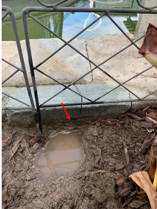
Photo No. 15: The crack continued across the top and back side of the pool wall. The water behind the pool wasn't a leak as some water was used to clean the concrete and expose the crack (red).
