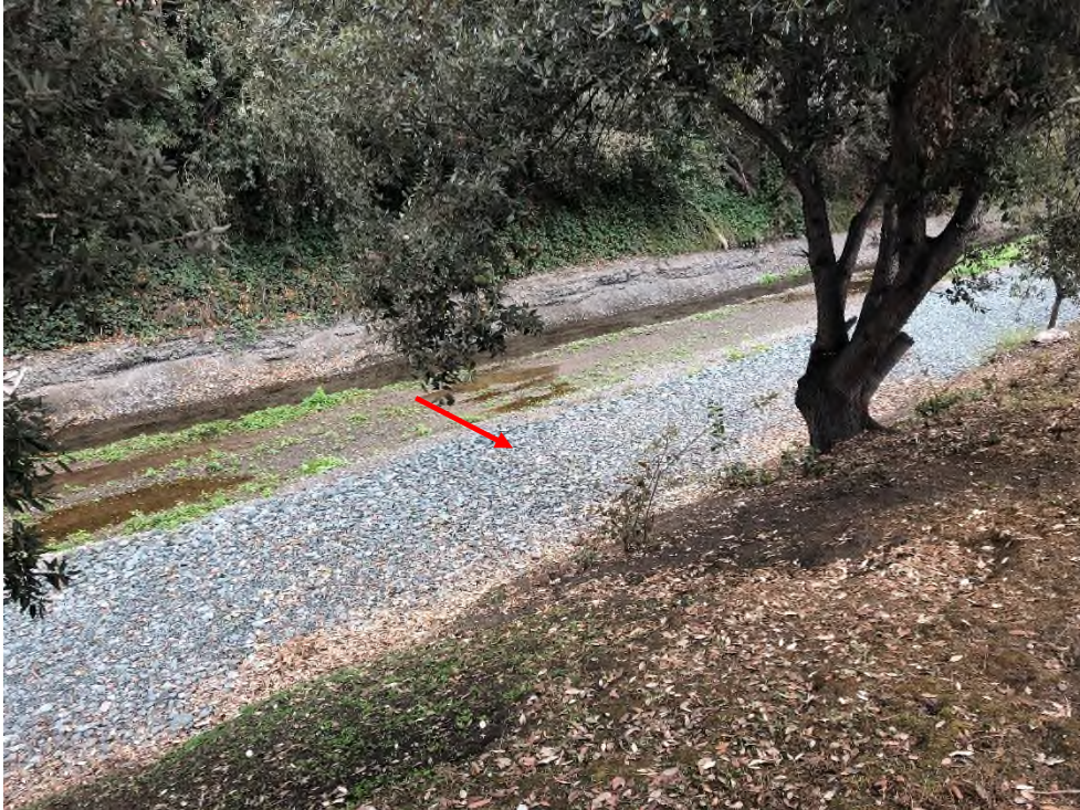
Photo No. 13: The gravel roadway (red), improved with heavy equipment including a vibratory sheepfoot roller, was almost 30' east of the claimant's pool. The gravel roadway was over 10' below the top of the bank.
