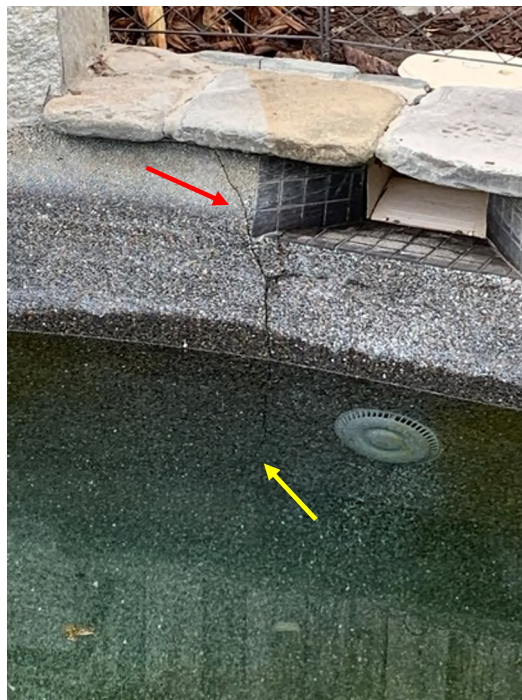
Photo No. 14: The pool was cracked in the shallow end. The crack extended several feet down the wall.
