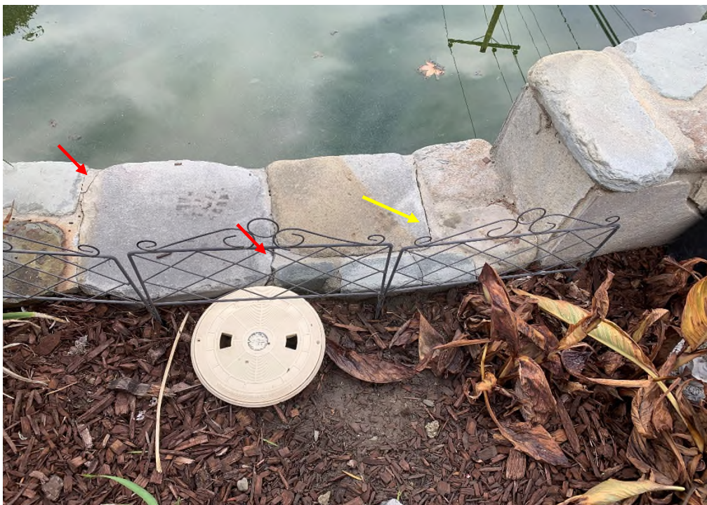
Photo No. 16: There were other cracks in the stonework besides the subject crack leading to the pool wall (yellow).
