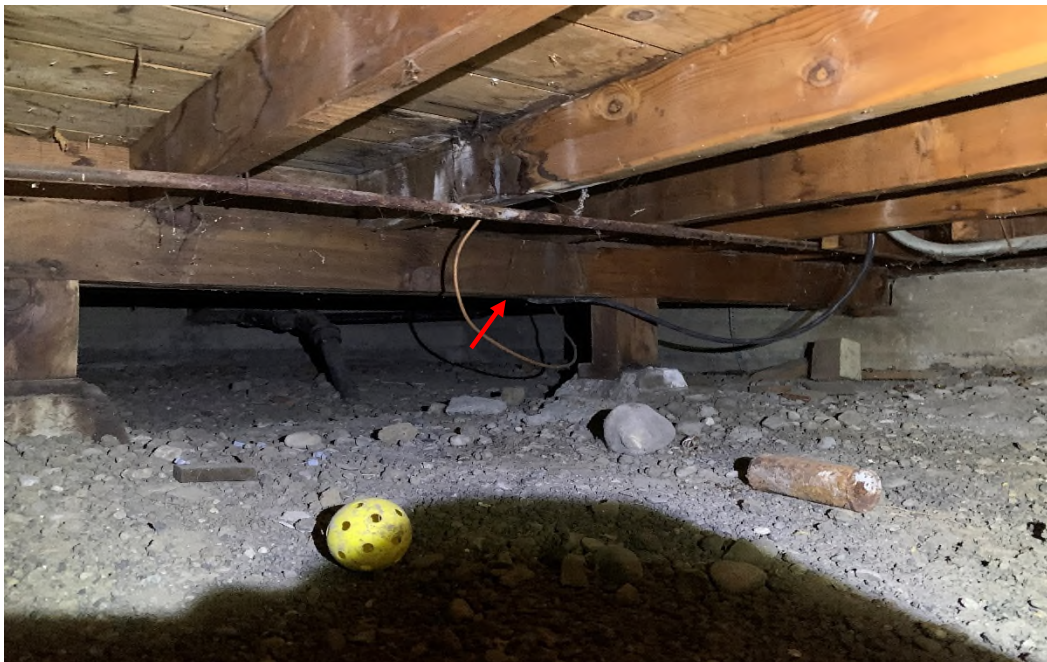
Photo No. 8: Below the kitchen, there was evidence of prior or current moisture exposure damage to framing and sheathing. The beam was visibly deflecting (red) along its span.
