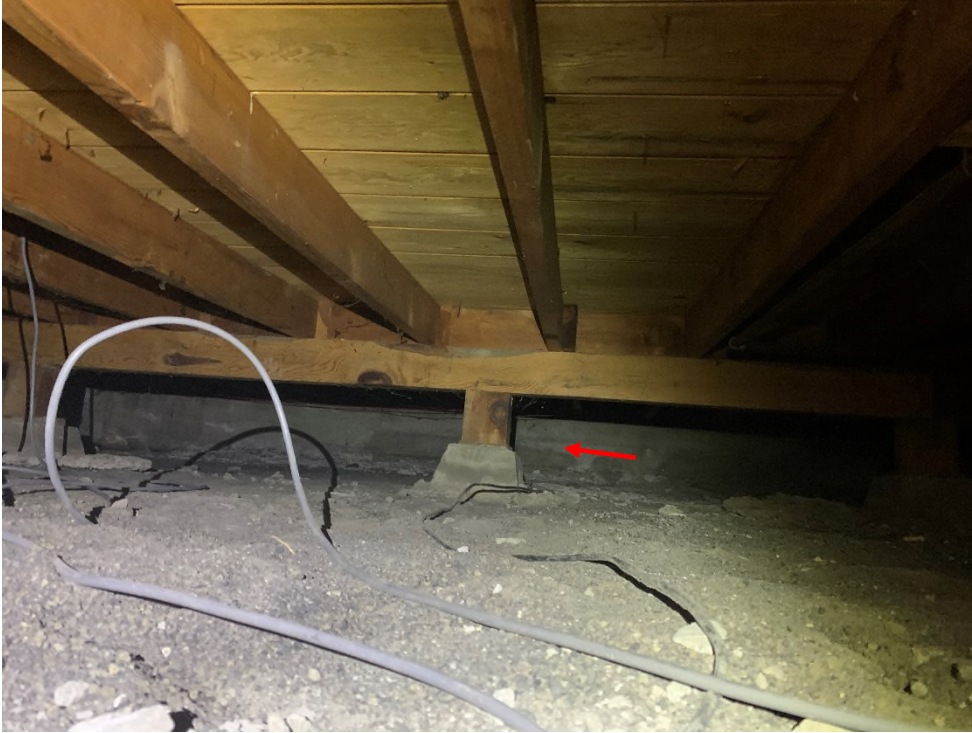
Photo No. 9: Concrete pier foundations had settled differentially into soil substrate. Posts were not plumb. Joists were not adequately connected to beams and unrestrained from rotation.
