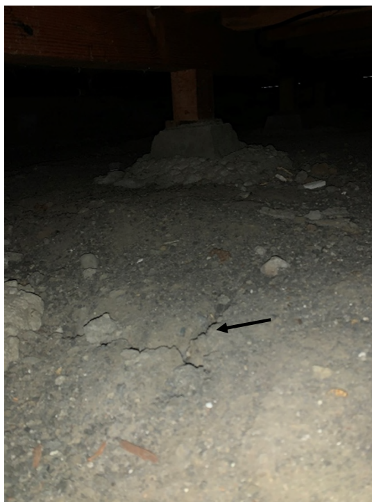
Photo No. 18: Large desiccation cracks in the crawl space soils indicated the presence of a clay element in the soils underlying the home.
