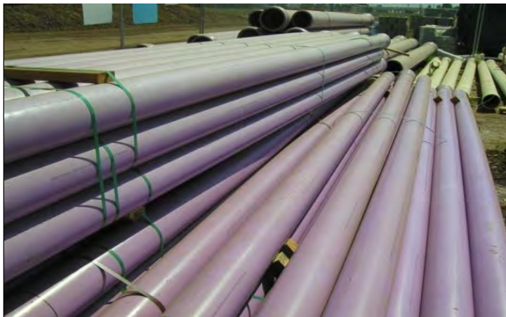
Purple recycled water pipe waiting to be laid during construction of the Immediate Term project
