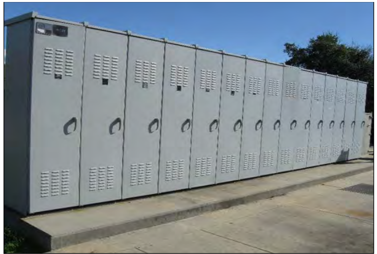
Motor control center switchboard
