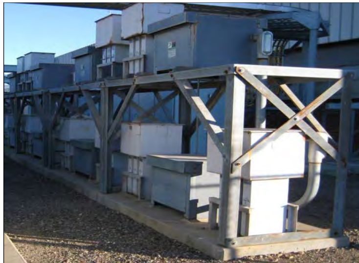
ASD motors at the Coyote Pumping Plant
