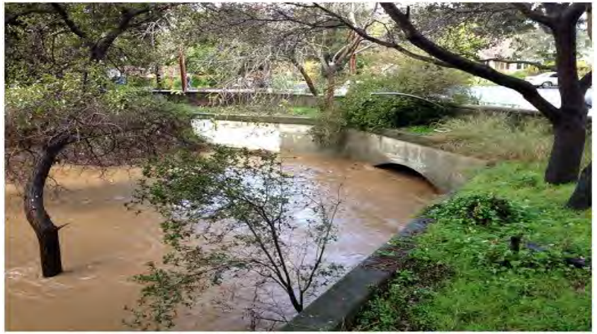
Upstream face of Pope/Chaucer Street with water surface approximately two feet below the soffit
