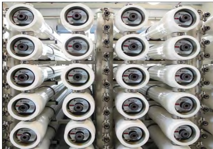
Reverse osmosis membranes used for water purification
