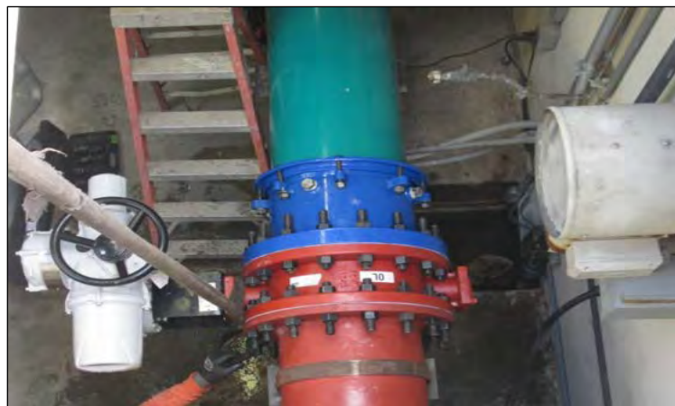
A typical rehabilitated line valve assembly
