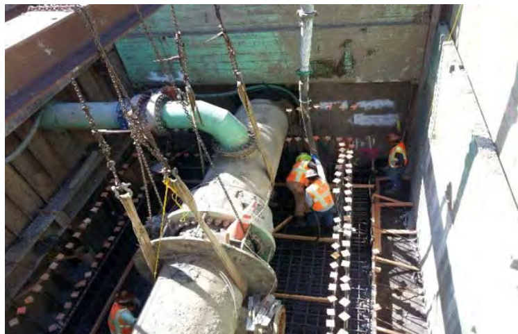
New interties similar to this will be installed in the cities of Santa Clara and Mountain View.
