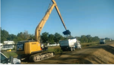
Sediment removal at Sunnyvale East Channel.
