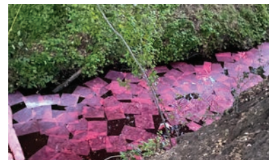
Absorbent pads soak up Matadero Creek diesel spill.
